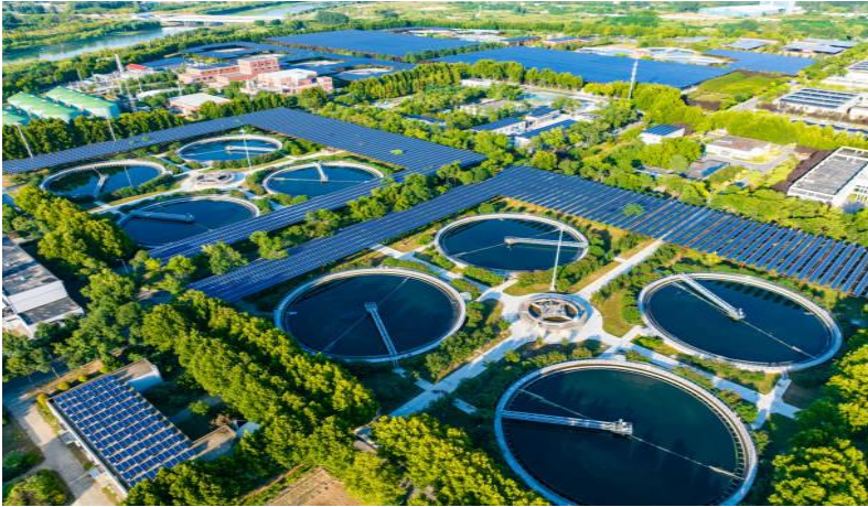
Solar Powered- Water Treatment Facility
